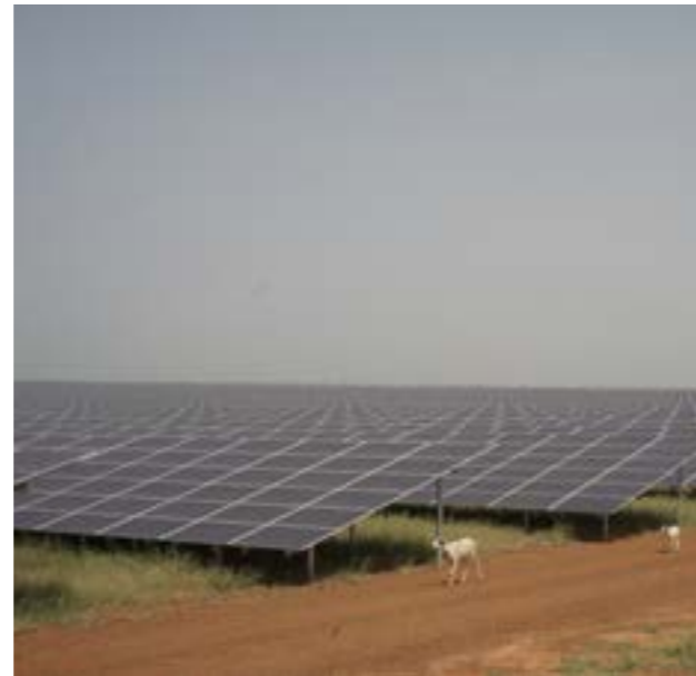
Senergy's photovoltaic solar power plant in Bokhol is the largest solar power station in West Africa.
